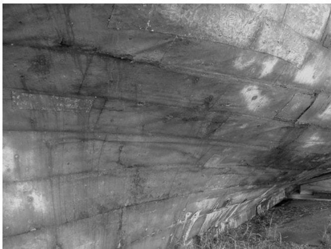
Figure 1. General view of copper sheathing in the hull of the Gades (Spanish Tug Boat, 1901)
