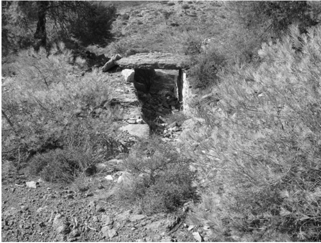
Figure 1. Rock walls conducted spring flow through a shallow channel into a shallow basin located just on the other side of the slab-covered portion
