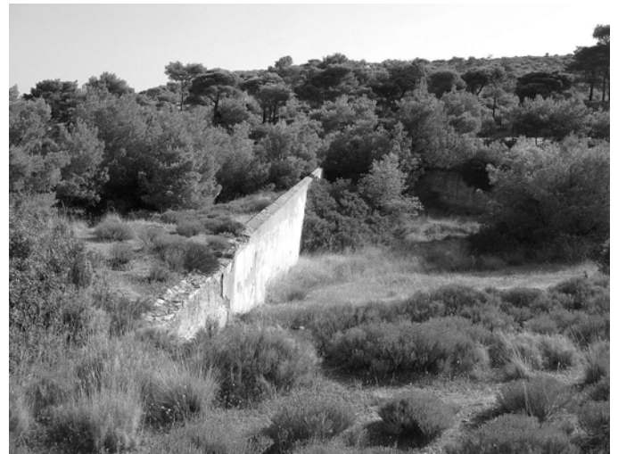
Figure 2. Ancient dam extends across a tributary valley to Camaresa Ravine. The south wall of the retention basin in the background runs along the south side of the thalweg of the tributary
