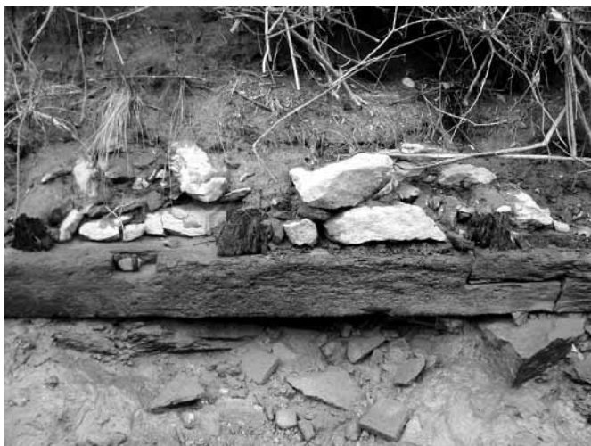
Figure 2. Timbers exposed at Falling Creek
